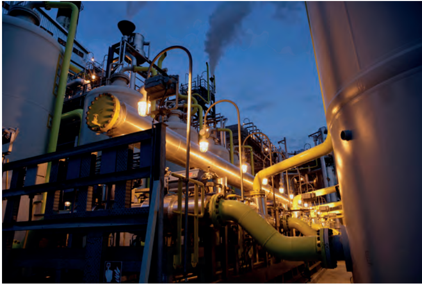
Fot. arch. PKN ORLEN
