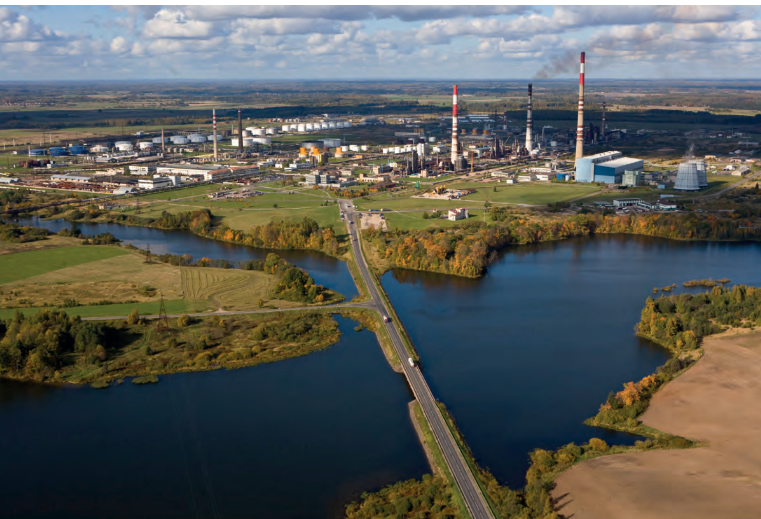
Fot. arch. PKN ORLEN
