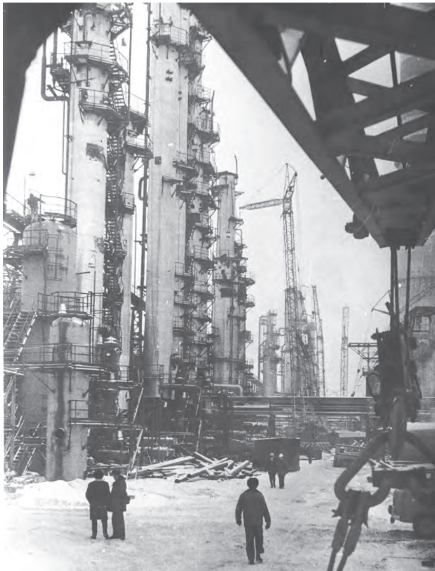
Fot. arch. PKN ORLEN
